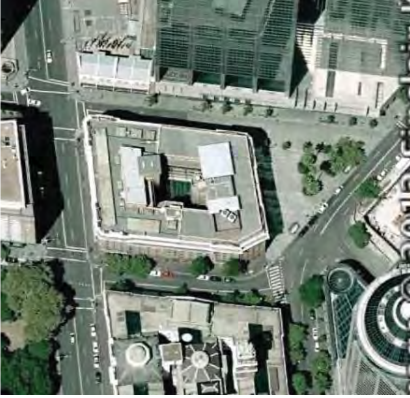
Existing condition: Farrer Place and surrounds
